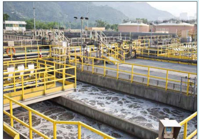
Waste Water Treatment Aeration Tanks
